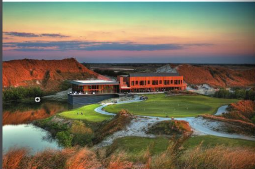
Streamsong Clubhouse viewed from the west.
